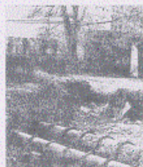
This cast iron water supply line was installed by Louis XIV of France in 1664. It's been in continuous service for over 325 years!
